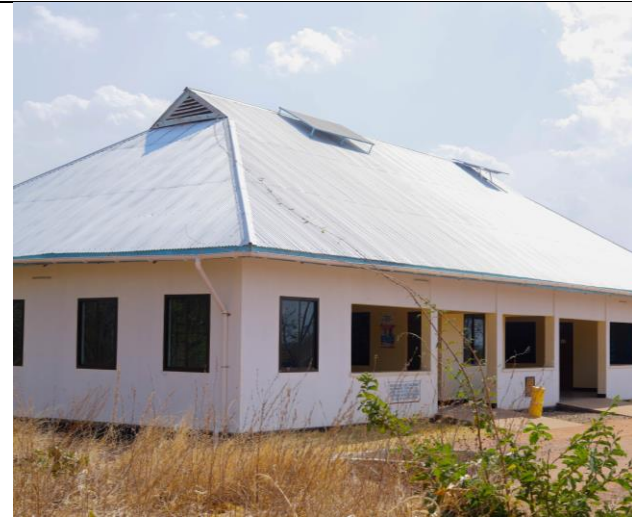
Kipunda village dispensary in Ikungi DC constructed by HAPA under Wibia e.V funding support-2022
